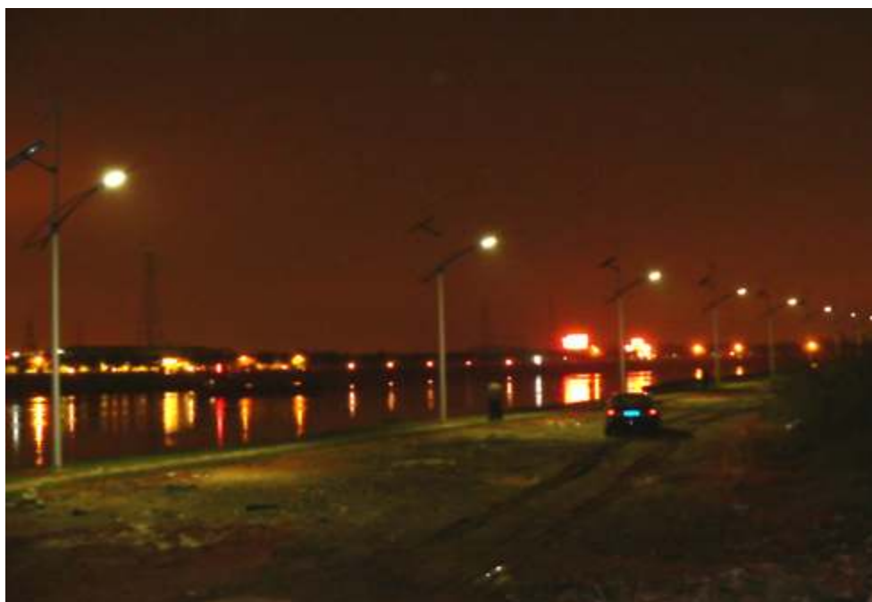
Night Scene, Roadside Wind/Solar Hybrid Lighting Power Supply System, International Bio-island.
